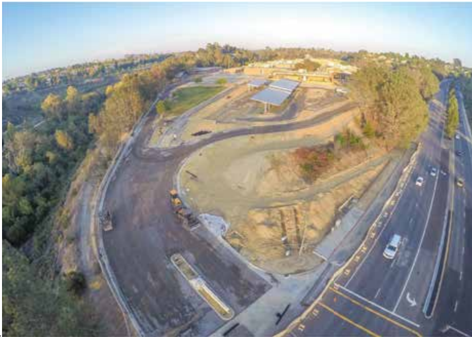
Aerial view of UC High School construction. Photo courtesy of Daniel Webber and Jack Gallegos.
