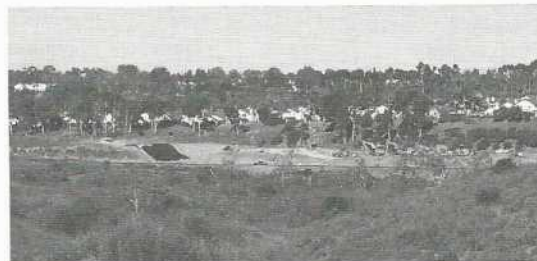
View of railroad project.
