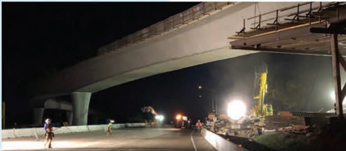
Crews wrap up falsework removals over southbound I-5 lanes
