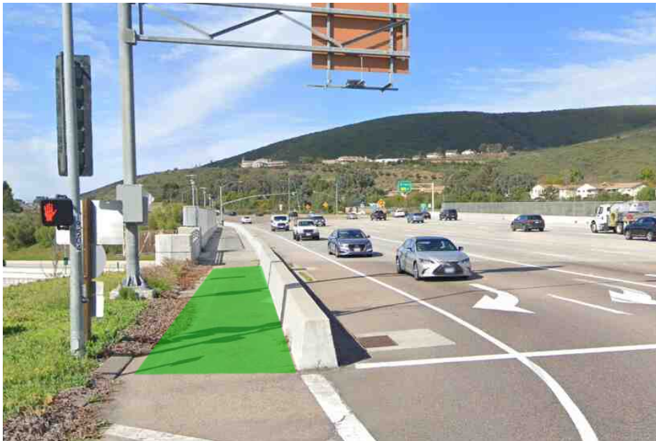
Example of Raised Concrete Barrier – SR- 56 over I-15
