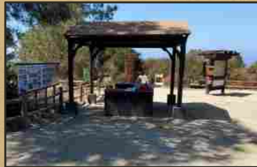
Non-compliant trailhead and kiosk
