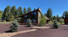
Defensible space works with well-maintained, fire-resistant vegetation.
